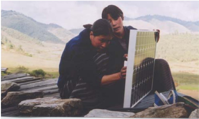
Local technicians install solar panel – Photo : Solar Electric Light Fund
